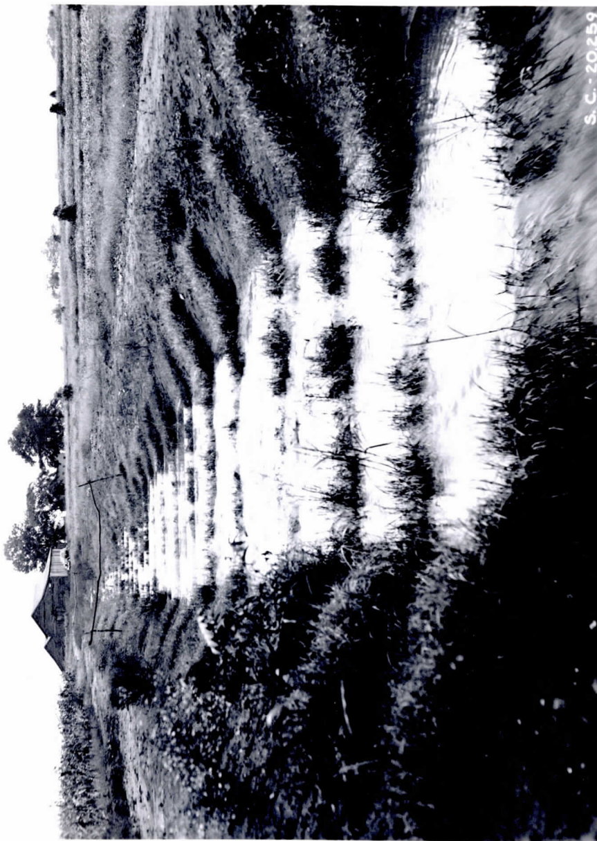
Figure 3 Bermuda Sod Terrace Out-let Channel on the T. C. Dunlap Farm. Note how well the Bermuda sod strips retard the flow of water. (Photo - Courtesy of Soil Conservation Service)
